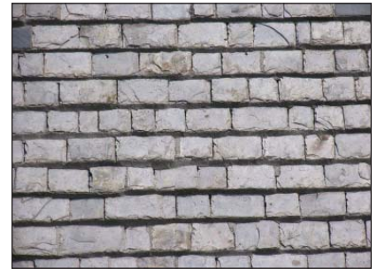
Distinctive local slate hanging
